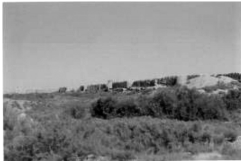
FIGURE 3 Sultan Kala City Walls, 8th century (Sayan, 1999).
