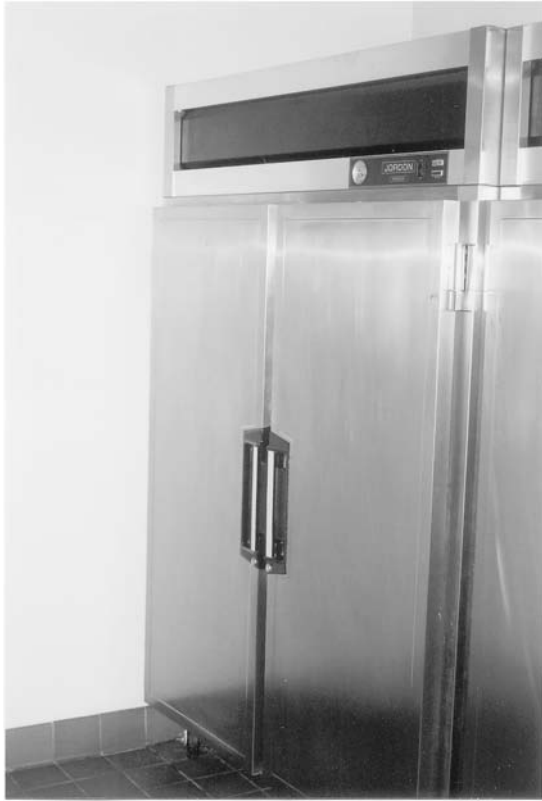
A reach-in refrigerator is used for storage of prepared food prior to service
