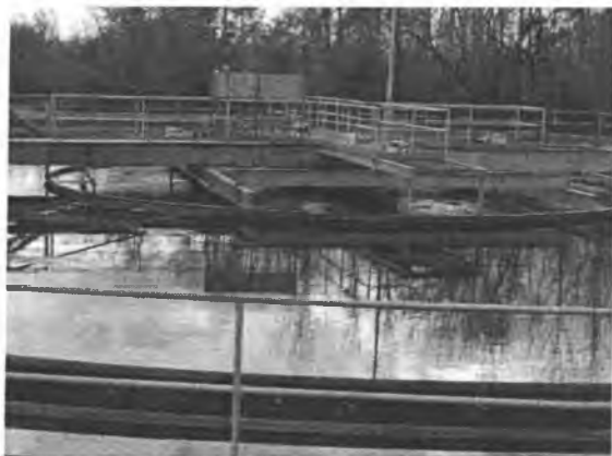
77-rasm. Ikkilamchi tindirgich.
