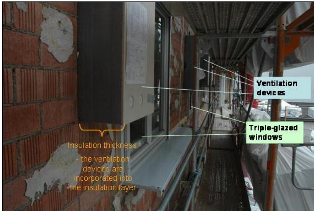
Figure 7.17: Refurbishment of the facade by triple-glazed windows, ventilation devices and 24 cm-insulation layer
