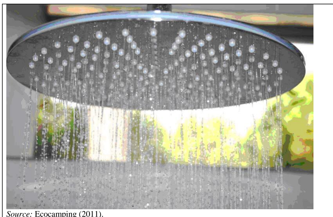
Figure 9.24: Example of a luxury low-flow rain-type showerhead installed in a luxury campsite, with a flow rate of 7 – 8 litres per minute
