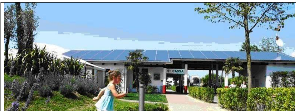
Figure 9.19: An example of solar PV cells integrated into a campsite building roof
